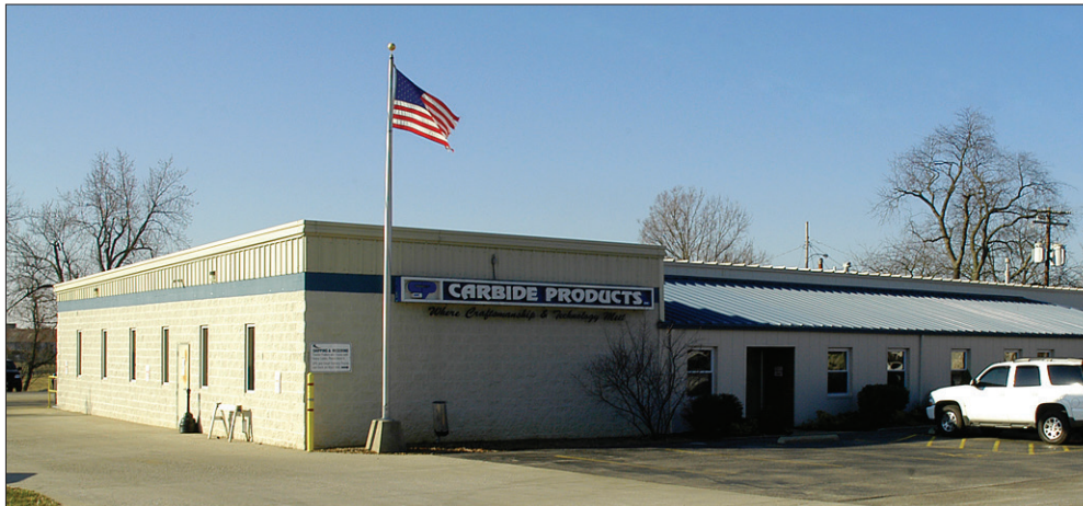
Carbide Products, Inc. makes use of an original structure built in 1958 as part of their 15,600 sq. ft. facility in Georgetown, KY.
