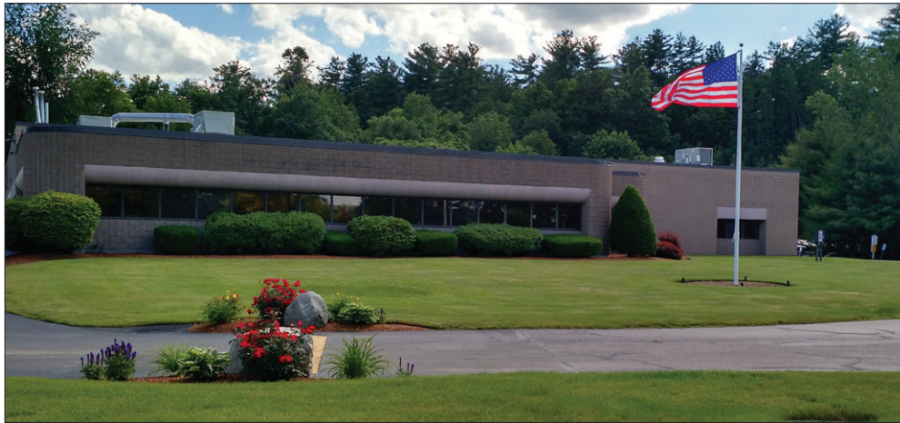
One of several buildings in the Kerk Products campus dedicated to manufacturing components for Haydon Kerk's line of precision motion control systems.
